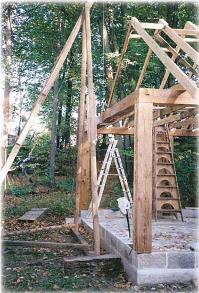
and to the vertical posts with countersunk 1/2" x 8" lag screws, which helps maintain a rustic appearance.
